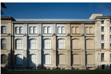
2 Diener Et Diener, New East Wing Expansion of the Museum of Natural History, Berlin, 1995-2010
