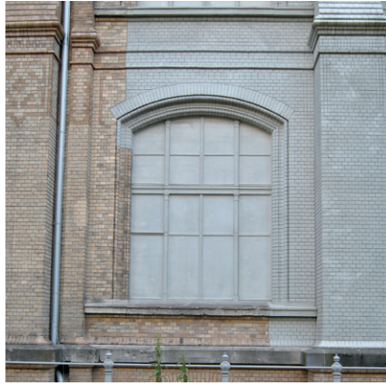
10 (left) Conversion of Convento das Bernardas, reinforced concrete windows
