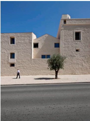
3 North façade of Convento das Bernardas
